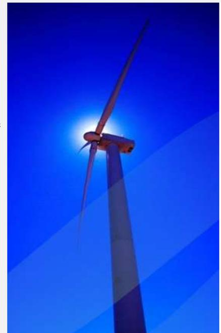
have the main rotor shaft and electrical generator at the top of a tower, and they must be pointed into the wind. Small turbines are pointed by a simple wind vane placed square with the rotor (blades), while large turbines generally use a wind sensor coupled with a servo motor to turn the turbine into the wind. Most large wind turbines have a gearbox, which turns the slow rotation of the rotor into a faster rotation that is more suitable to drive an electrical generator.
